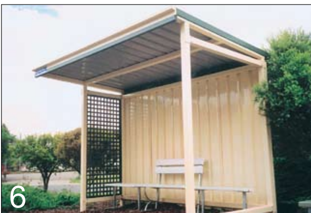
• Flat Roof Shelter
