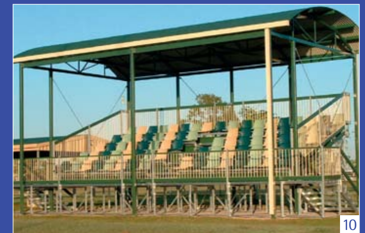
10 Rolled roof shade structure & tiered seating grandstand
