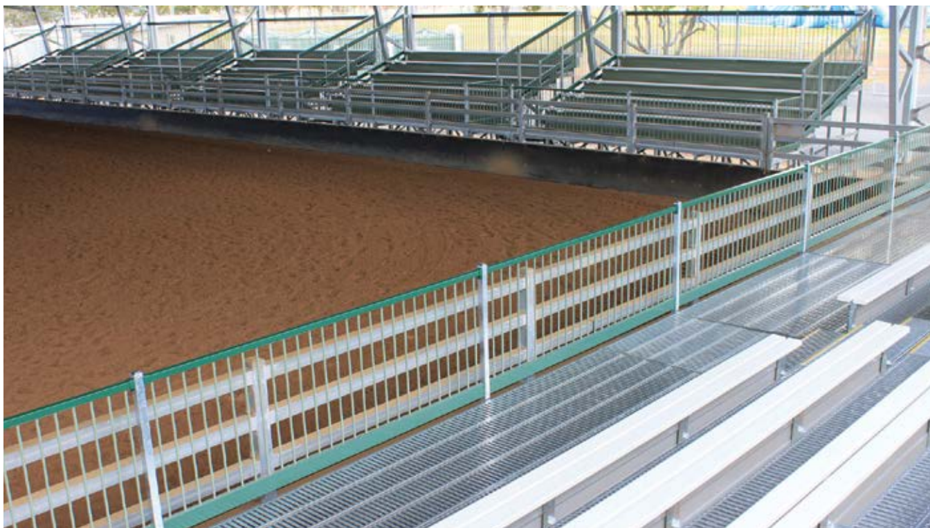
BUNDABERG SHOW GROUNDS: RAISED DECK BLEACHER SEATING
