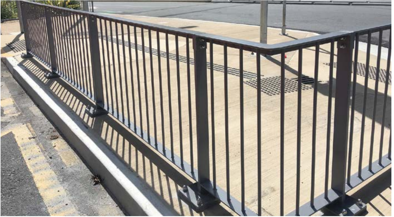
GOLD COAST LIGHT RAIL – ROAD SAFETY BARRIER FENCING; INSTALLED FOR BMD AS PART OF THEIR DELIVERY OF THE LIGHT RAIL INFRASTRUCTURE.
