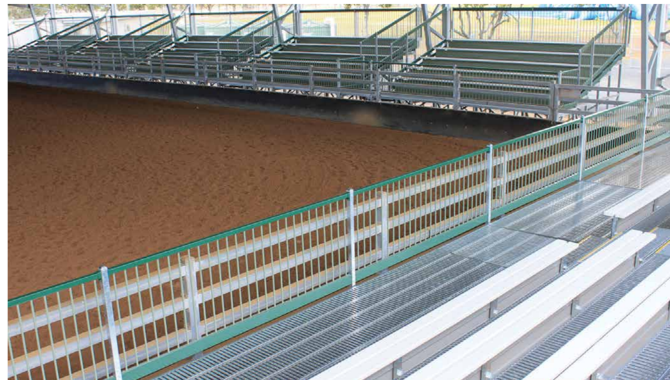
BUNDABERG SHOW GROUNDS: RAISED DECK BLEACHER SEATING
