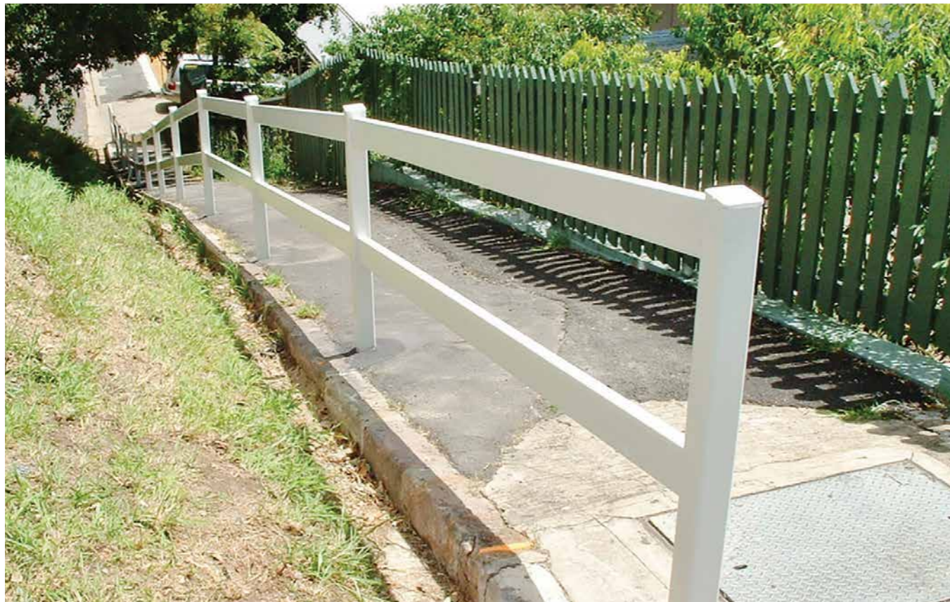
Council fencing – our square & rectangular colorbond locsteel looks like heritage hard wood timber fencing with the maintenance free & longevity of colorbond steel. This fencing is used extensively in by Brisbane city council & local government areas across Sydney city
