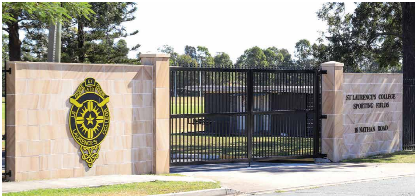
SCHOOL SPORTS FACILITY - ENTRY WALLS & AUTOMATED SECURITY GATES
